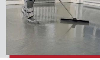
Cemfloor FSC 515 Smooth is a pump applied, self smoothing thin topping compound for floors which gives a strong surface layer for early floor covering. The product is formulated from special cements, aggregates and chemical admixtures.
