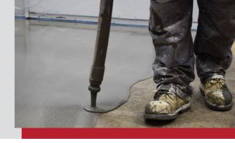
Cemfloor FSC 516 Rapid is a pump applied, rapid drying, self smoothing compound for floors, which gives a strong surface layer for early floor covering. The product is formulated from special cements, aggregates and chemical admixtures.
