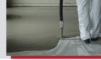
Cemfloor FSC 531 Fibre is a pump applied, self-smoothing, fibre-reinforced base or renovation screed for floors which gives a strong base layer for receiving tiles or a thin topping screed. The product is formulated from special cements, aggregates and chemical admixtures.
